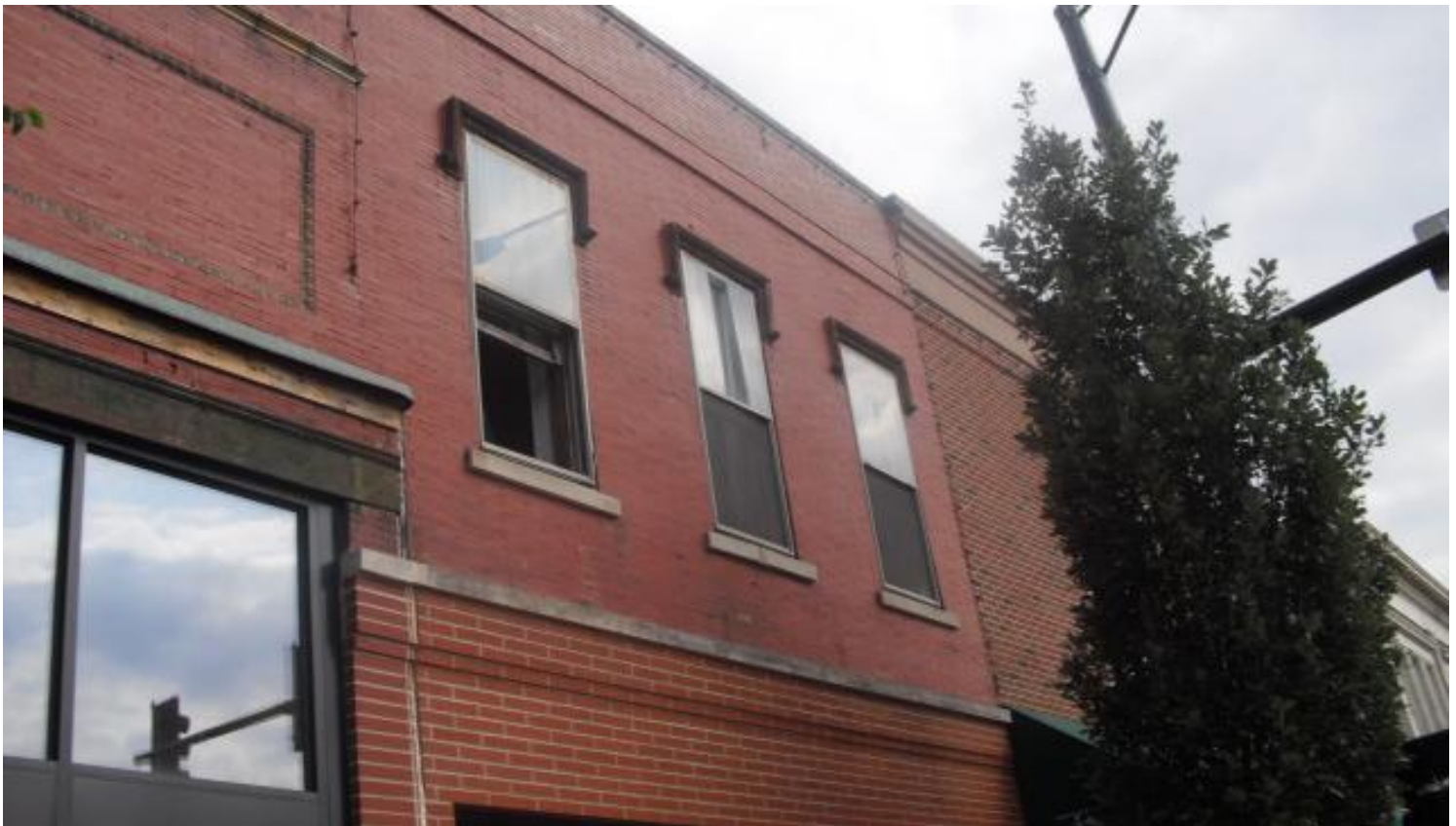
Photograph #1: South Wall Second Story
