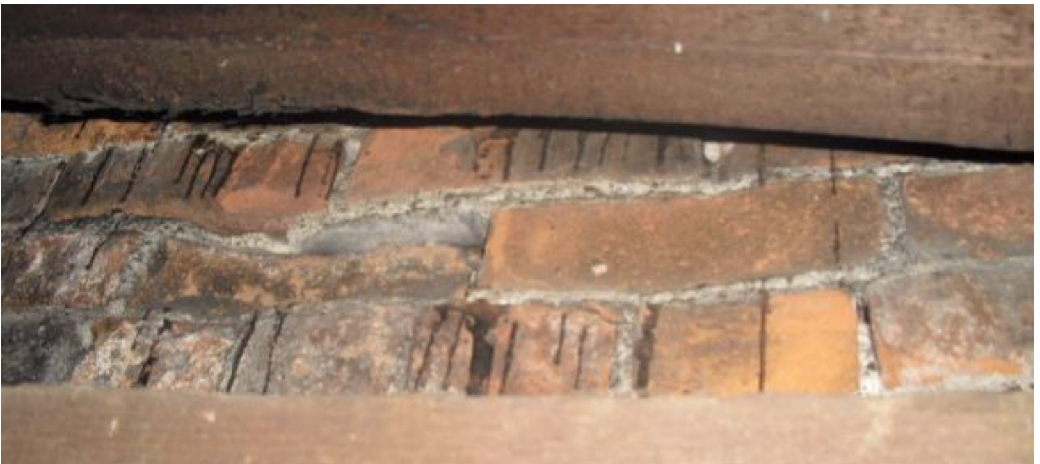
Photograph #3: Poor condition of Interior Brick Wythe, east end of South Wall
