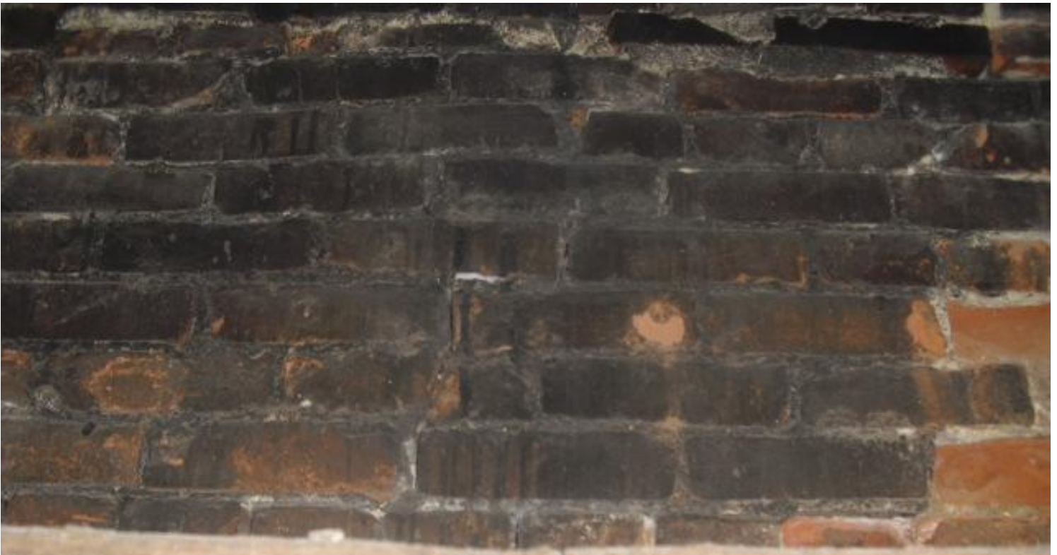
Photo #5: Deteriorated Interior Brick Wythe and Water Penetration Evidence
