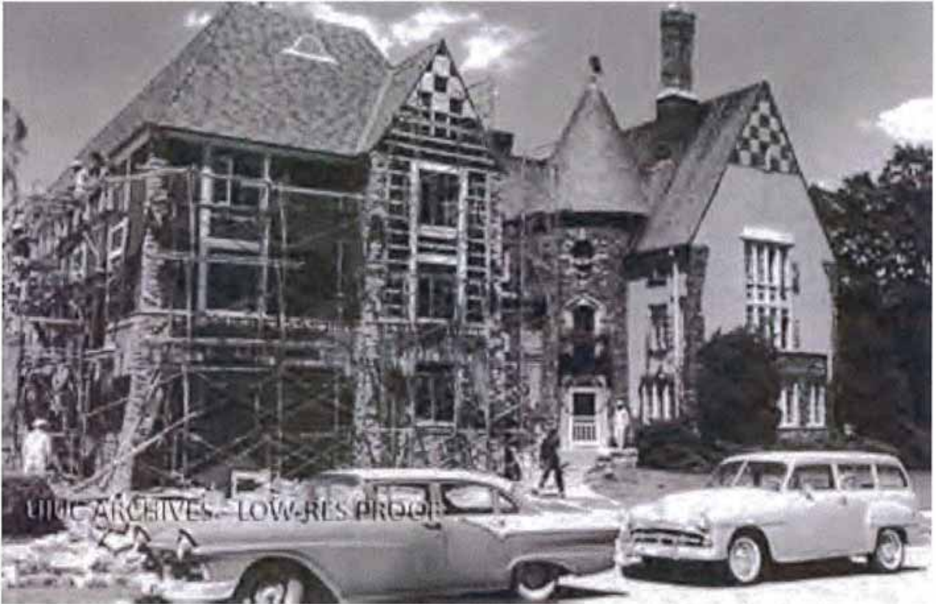
Zeta Tau Alpha House Addition Under Construction, 1962
