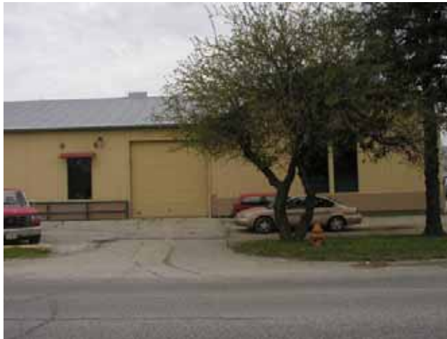
TK Service Center, mid-section of building along Perkins Rd
