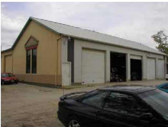
TK Service Center, east portion of building along Perkins Rd and east elevation of building
