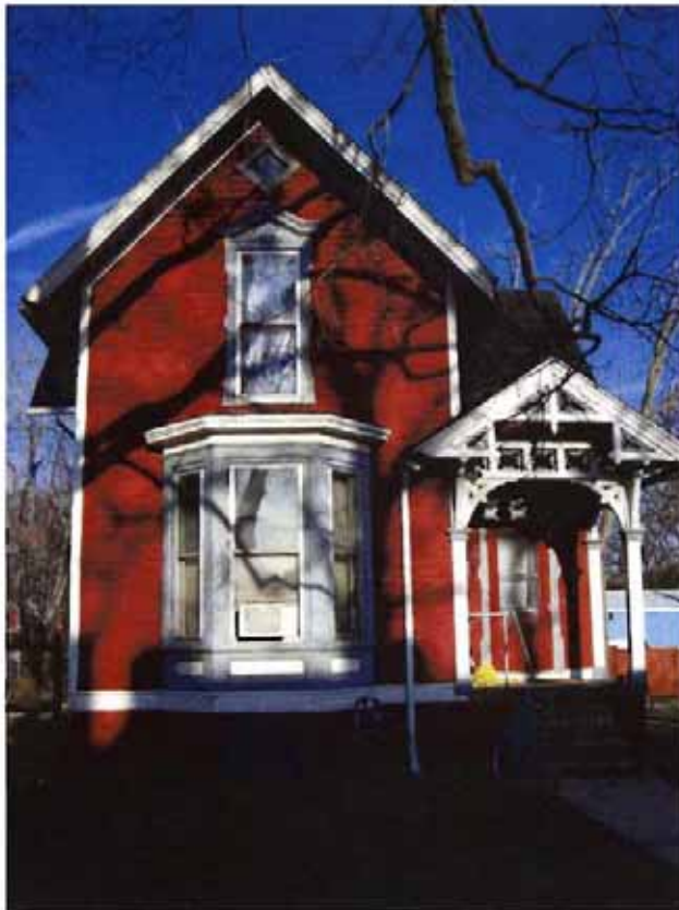
View of west elevation.
