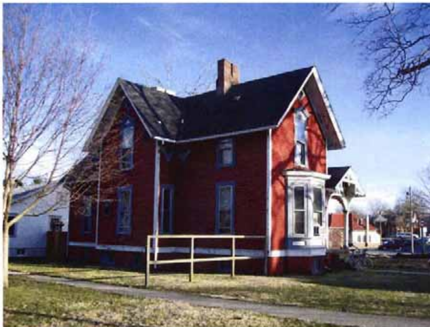
View of north and west elevations. View is towards the southeast.
