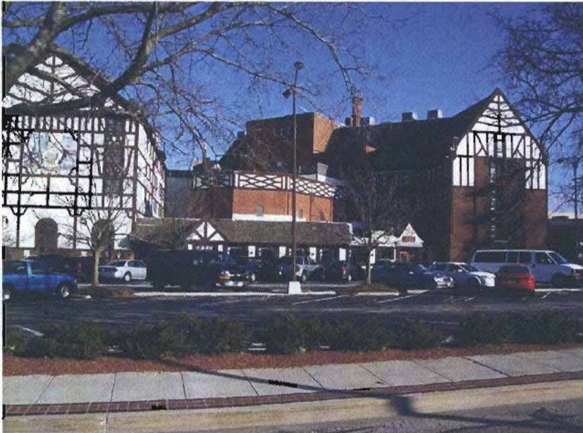
Current west entrance
