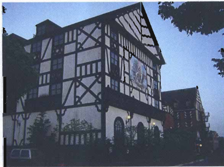
1980s addition, west facade
