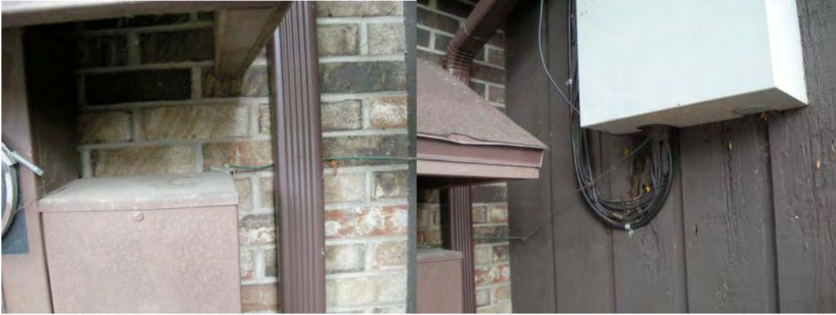
511 S. Elm; Multiple Dwelling Unit; ground OK.
