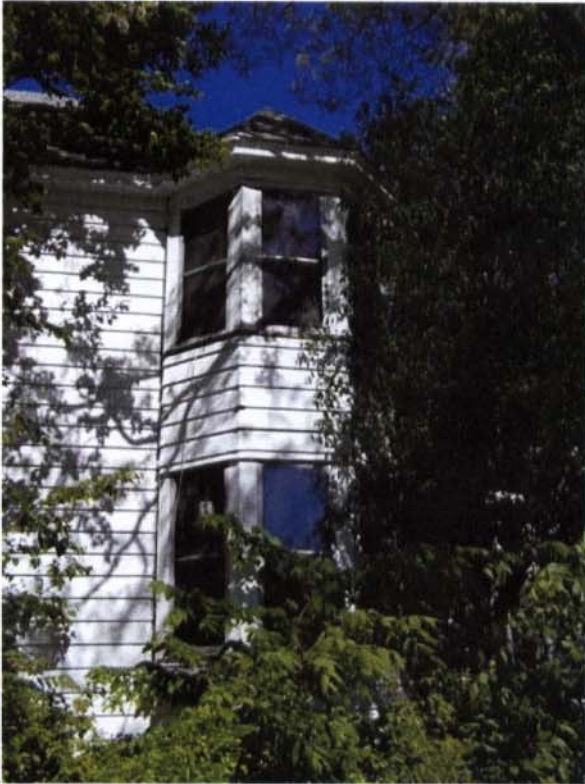
508 West Elm Street. Southwest corner tower.
