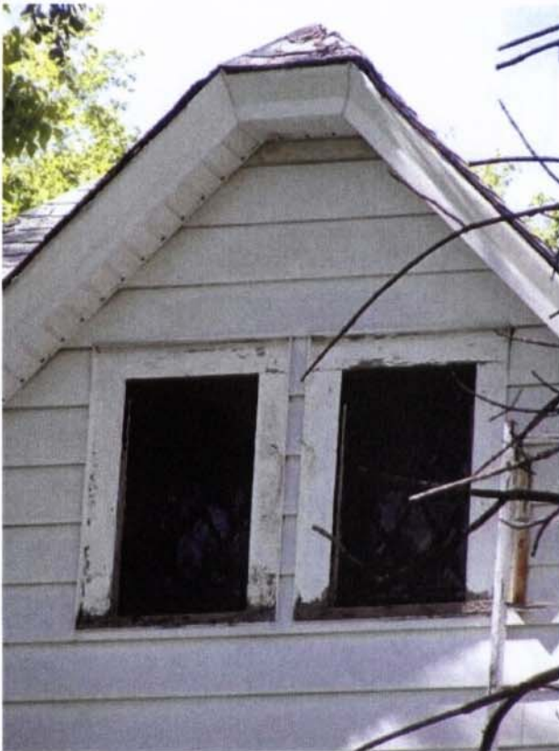
508 West Elm Street. South elevation, clipped wall gable with diamond/lattice casements.
