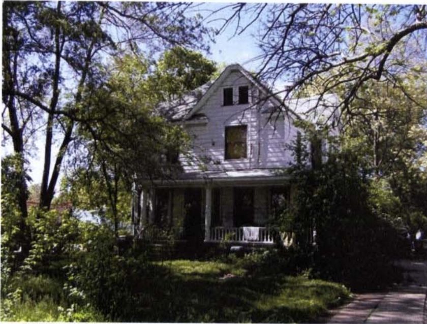
508 West Elm Street. South elevation
