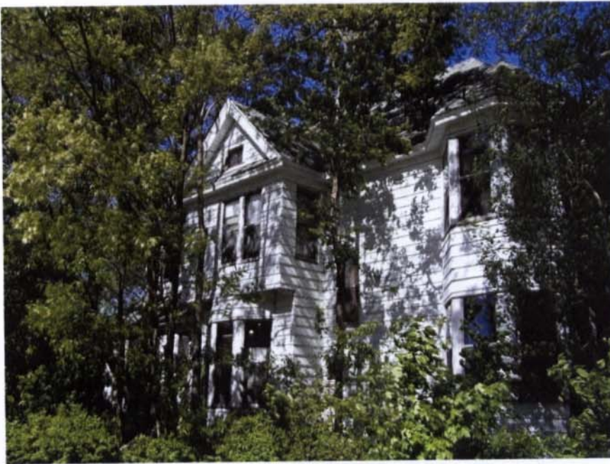
508 West Elm Street. West elevation.
