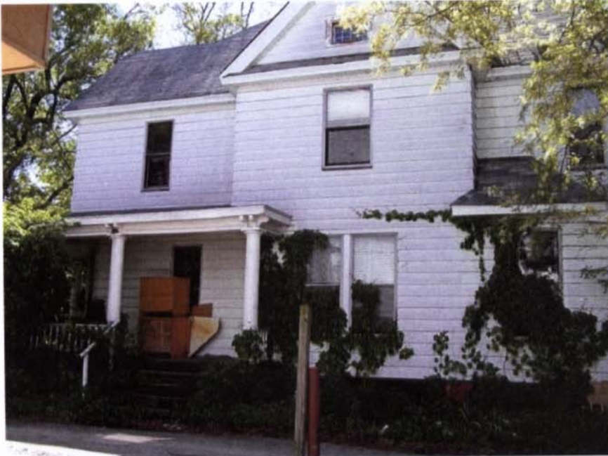
508 West Elm Street. East elevation.
