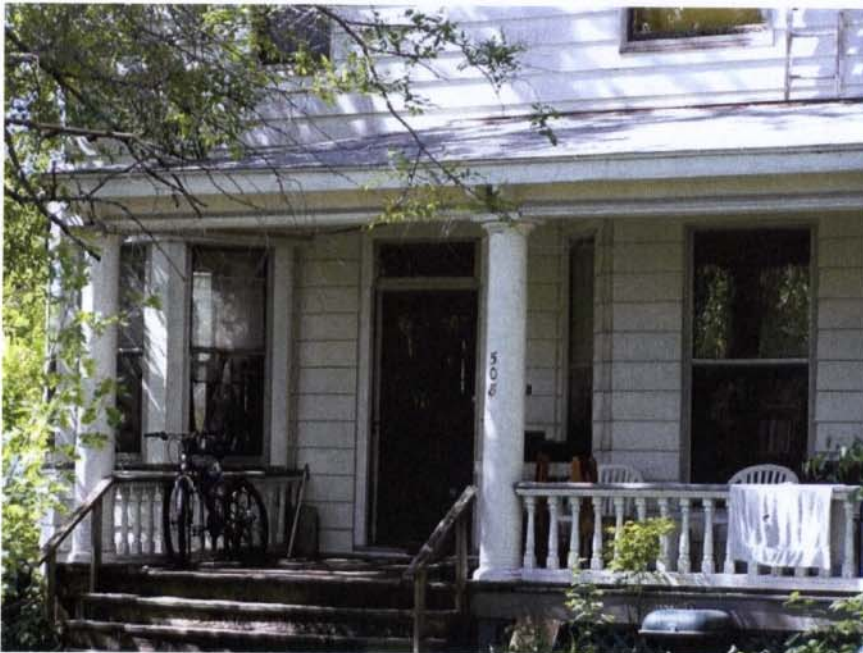
508 West Elm Street. South elevation, porch detail.
