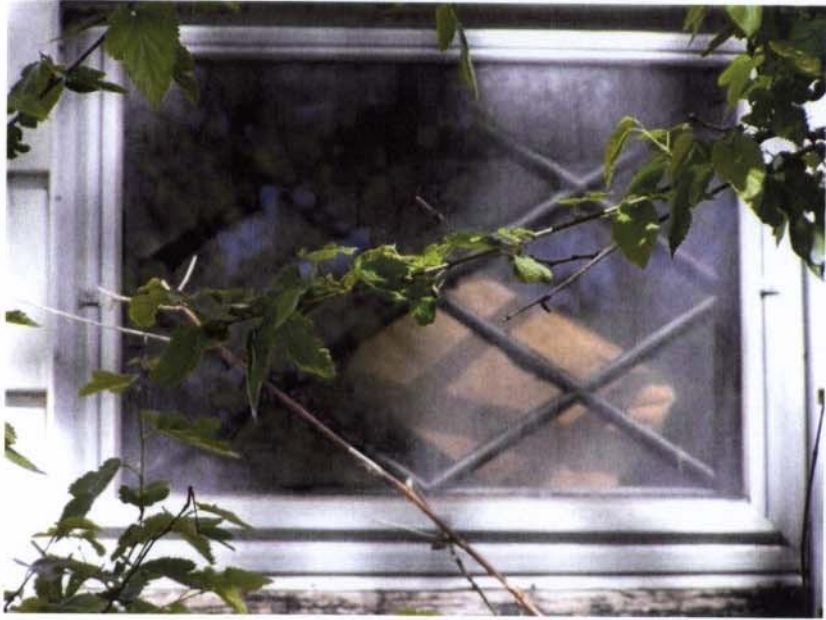
508 West Elm Street. West elevation, diamond/lattice-paned glass window.
