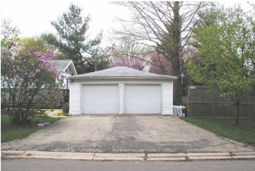
Looking west at existing garage from Broadway. The Bald Cypress is to the right of the garage.
