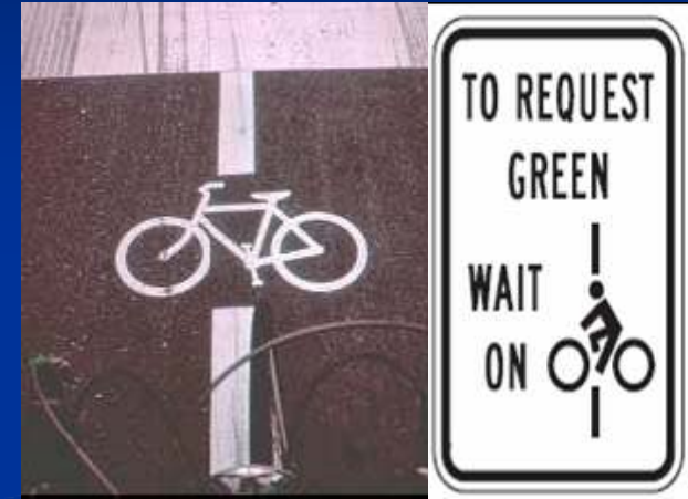
Signal activation marking and sign
