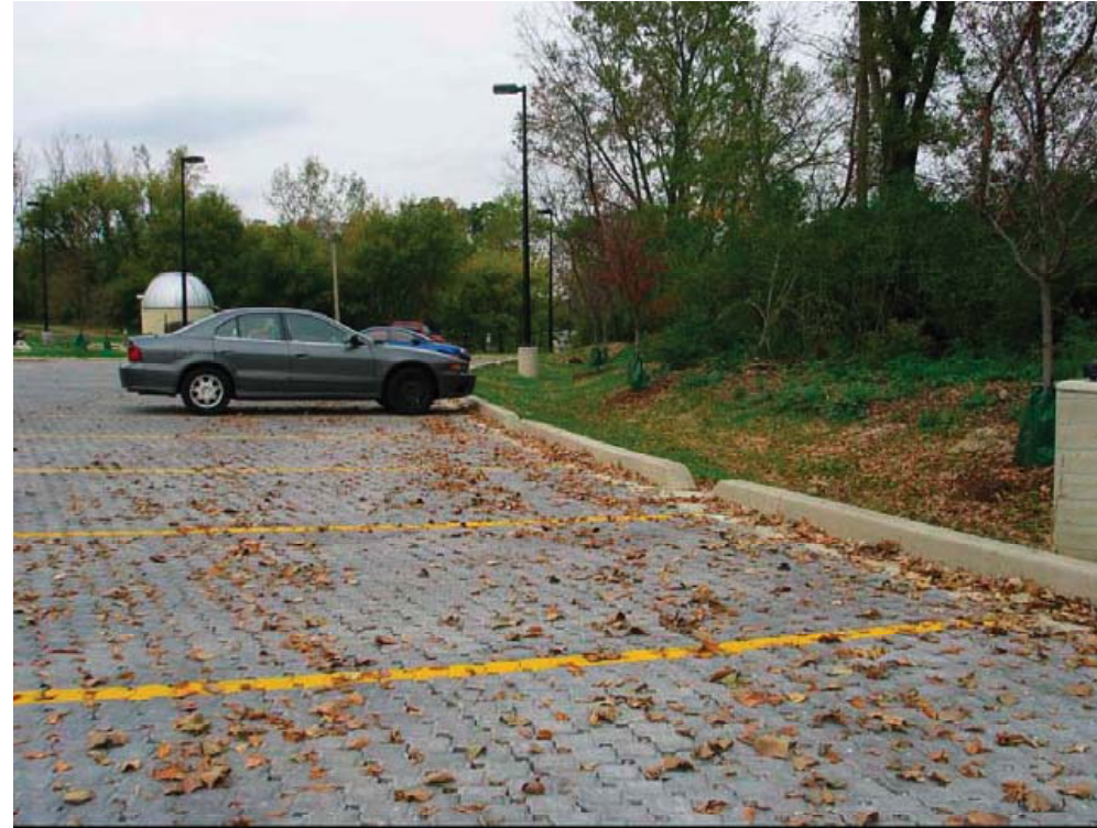
Pervious paver parking lot.
