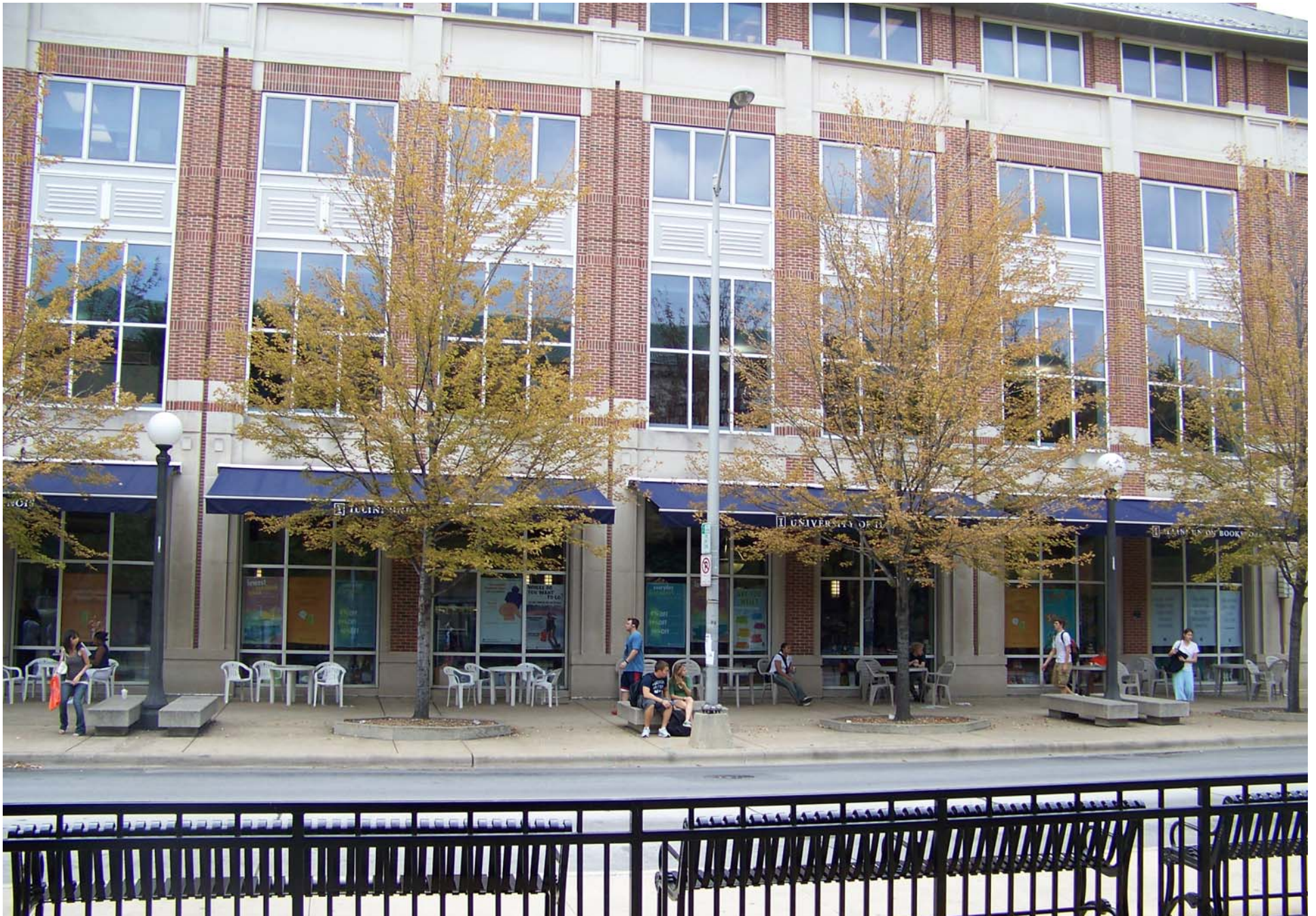
Existing– Wright Street Lights
