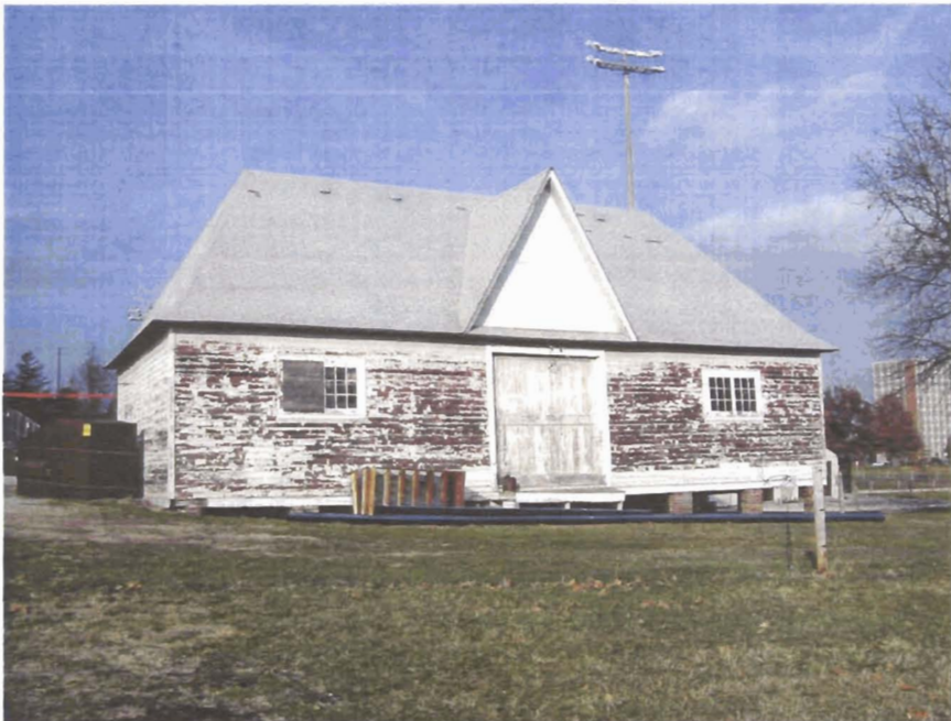
Mumford Horse Barn (facing north)
