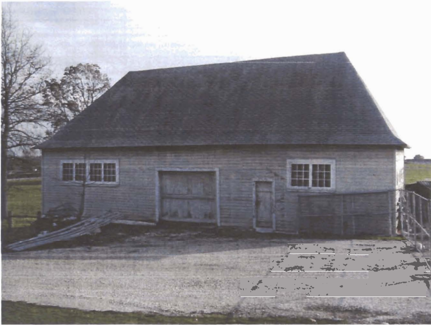
Mumford Horse Barn (facing south)
