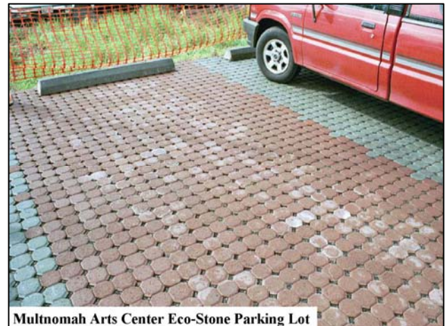
Multnomah Arts Center Eco-Stone Parking Lot
