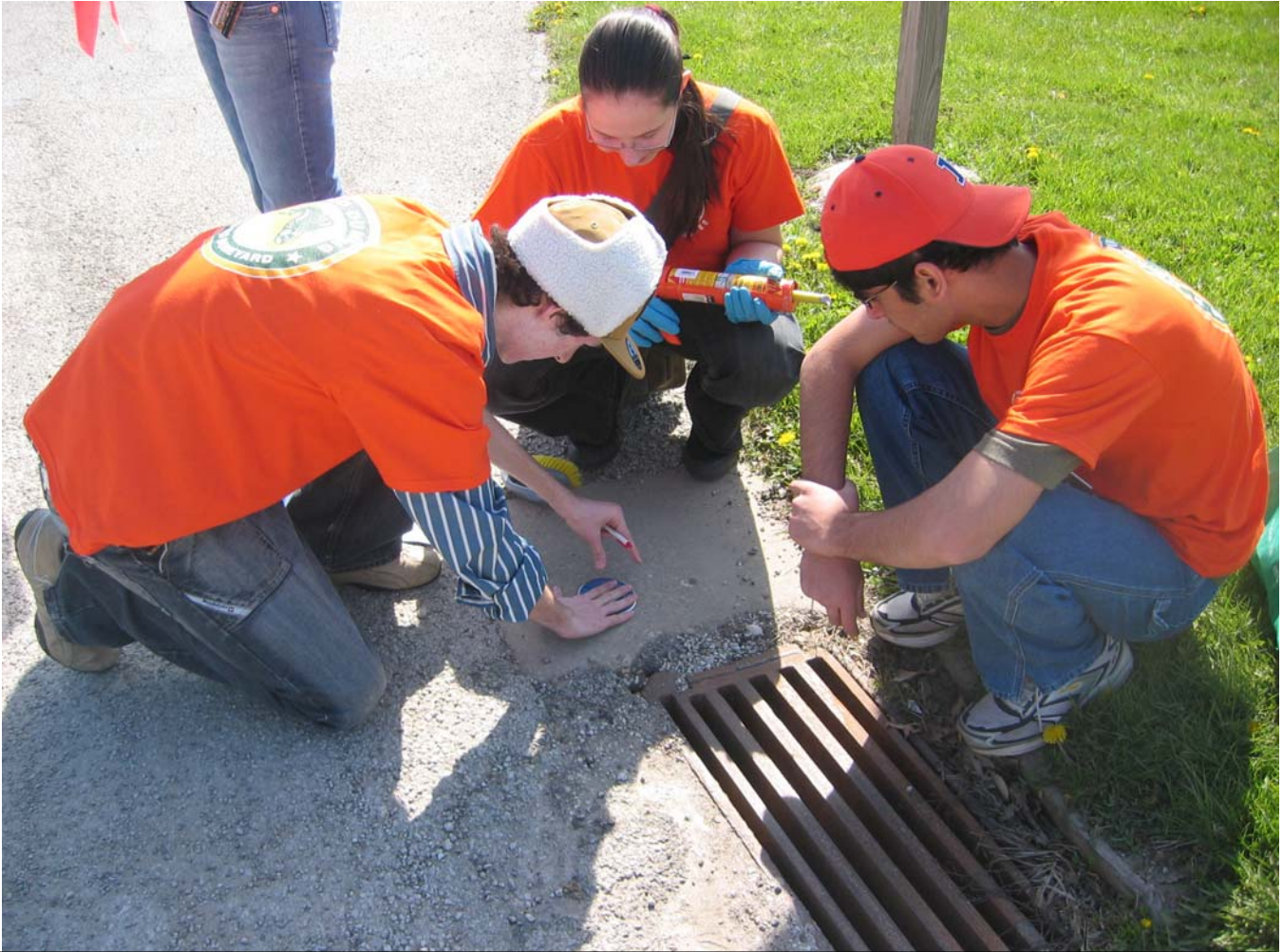
Storm Sewer Inlet Medallion Installation
