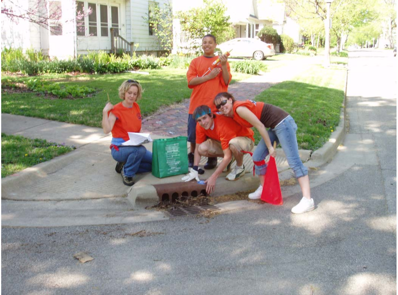
Storm Sewer Inlet Medallion Installation
