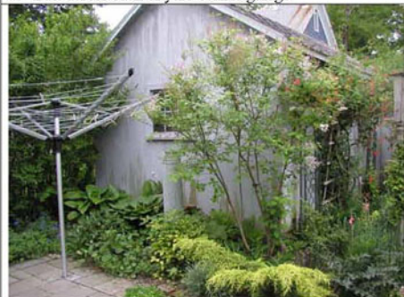
#9 North face of garage
