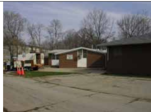
D. Don Moyer - Lakeside Terrace @ Bend facing Northwest.
