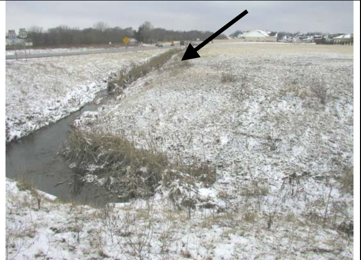
#2 View west from edge of Rt. 130 pavement
