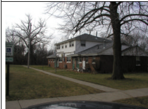
E. Lakeside Terrace at Don Moyer facing South.
