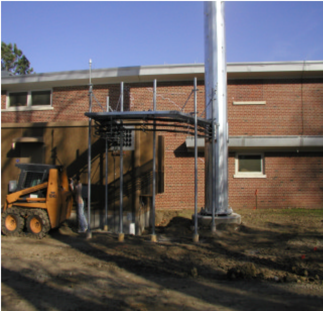
Cell Tower Site-Facing East
