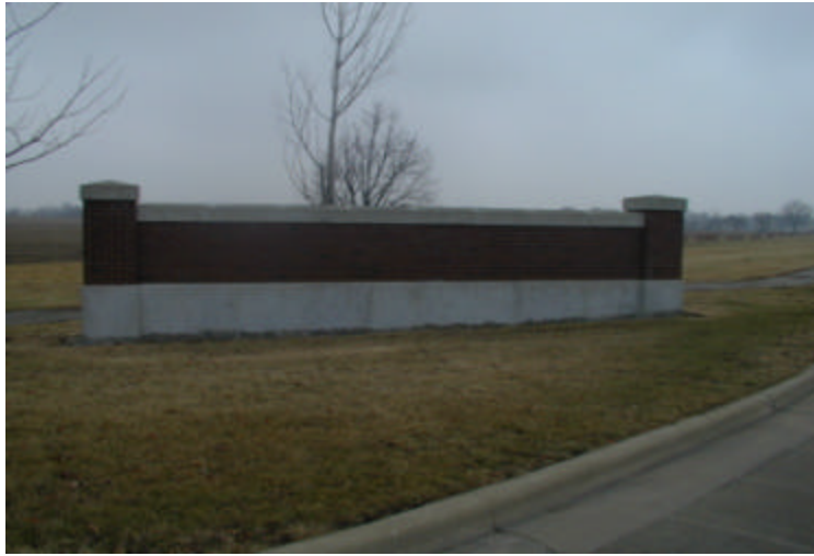
U of I Entrance Project On The Northwest Corner Of Windsor And Race In Urbana
