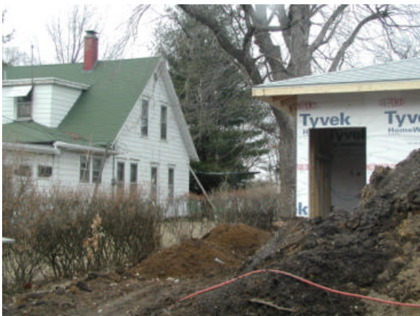
View from the rear alley
