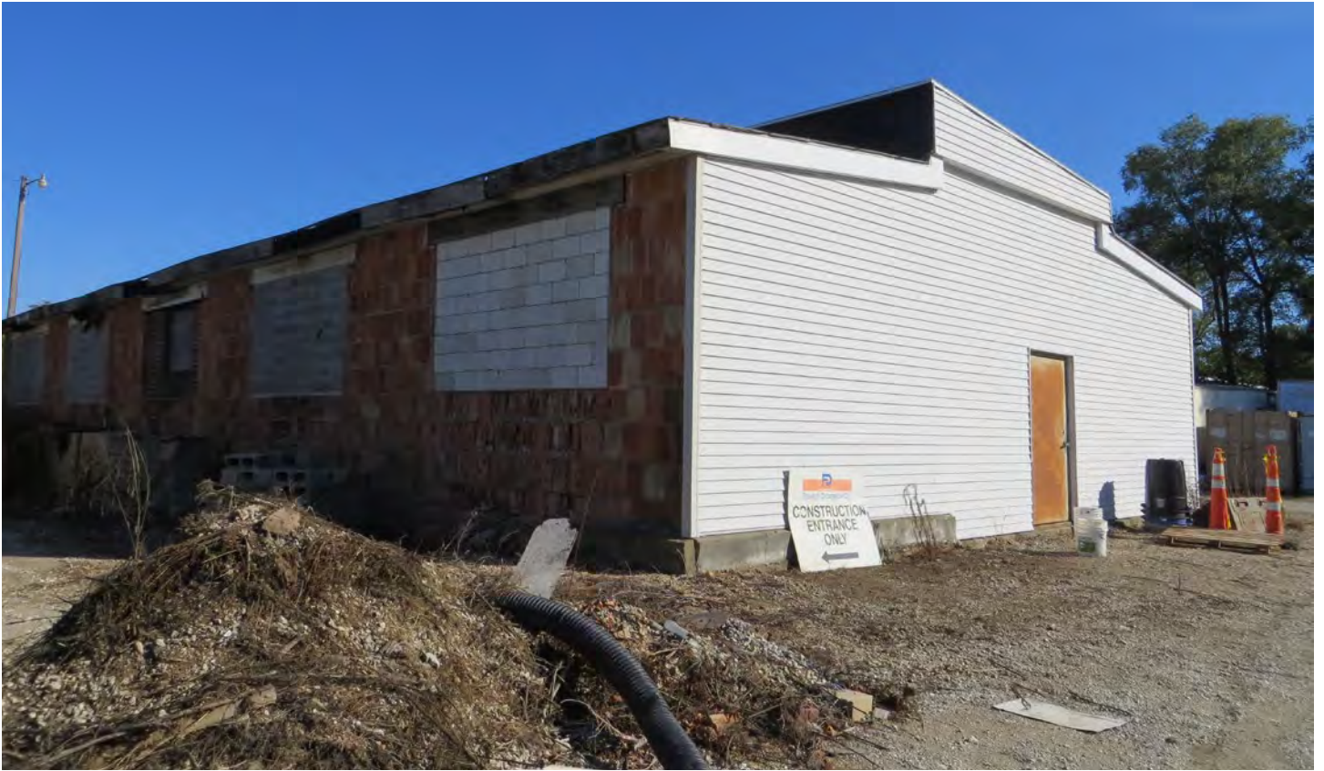
Existing warehouse proposed to be replaced
