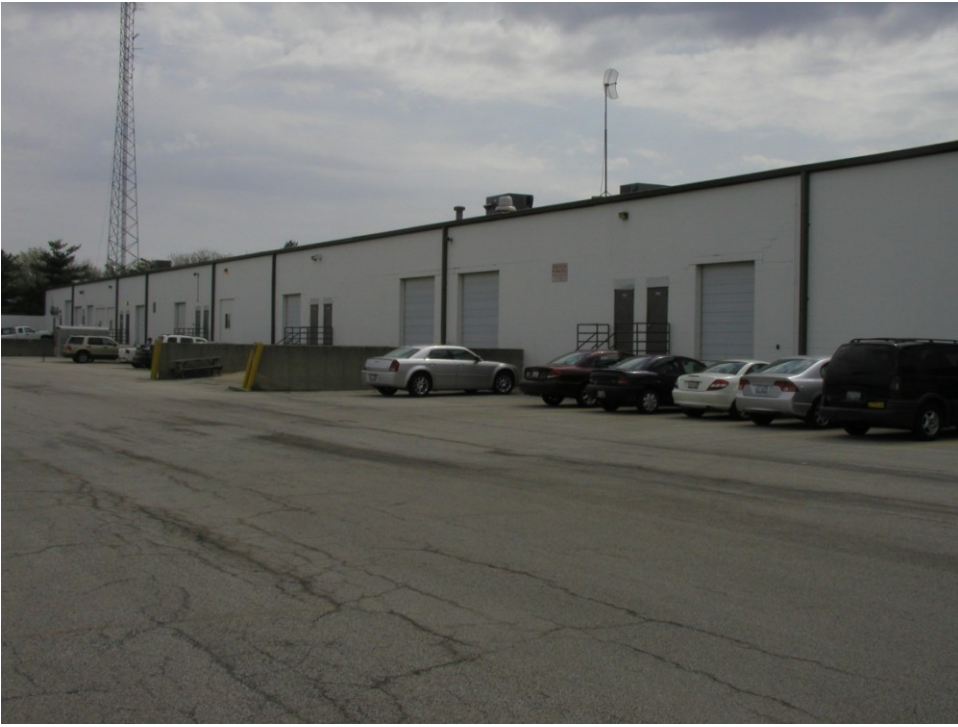
Figure 3. Lincoln Commerce Center, rear façade, loading docks & parking
