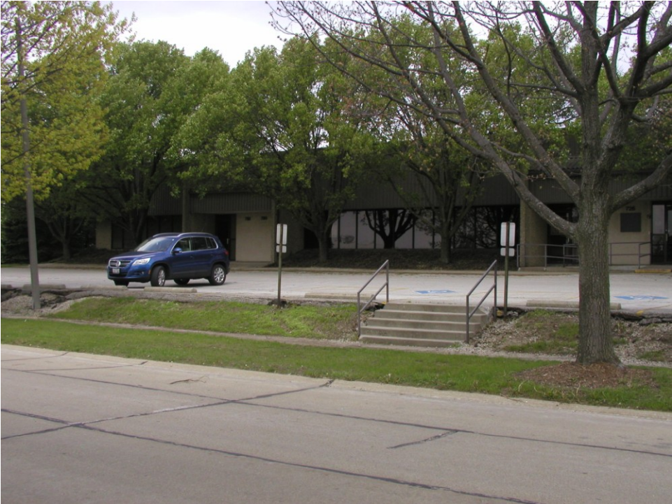
Figure 1. Lincoln Commerce Center, front facade
